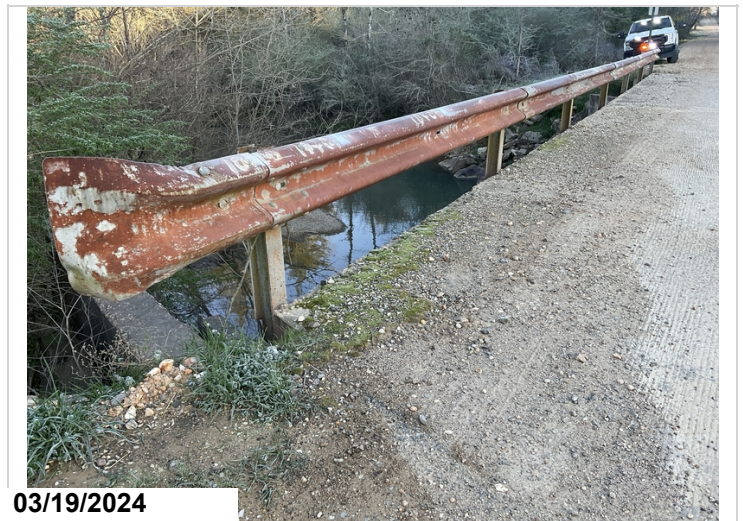
Lt side metal bridge railing, Minor corrosion, Typical of both right and left sides
