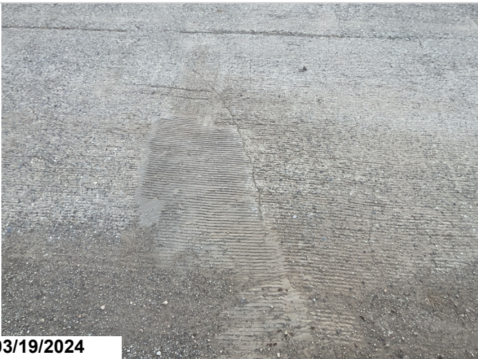
Rt side of bridge deck, Deck cracking, Typical in various locations.
