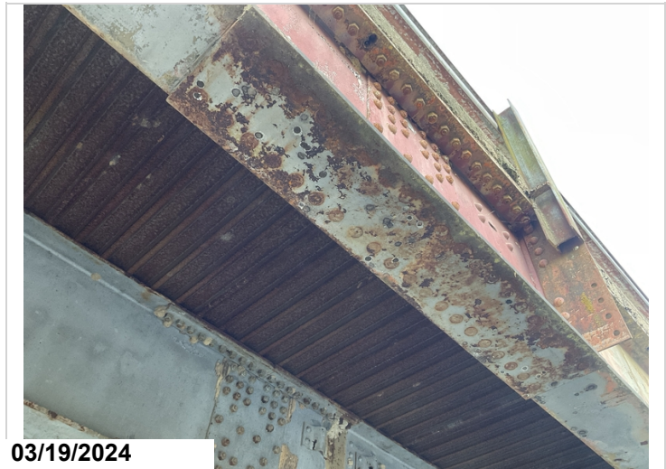
Beam 5, Minor corrosion, Typical throughout all beams
