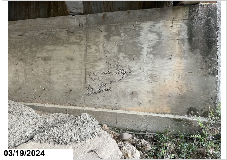
Abutment 2, Rt side, Honeycomb area, Typical in various locations of both abutments
