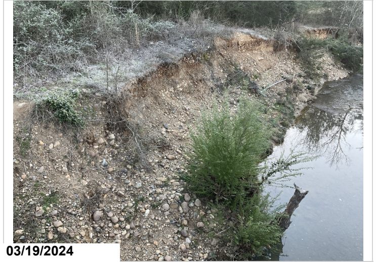
Downstream embankment damage
